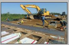
Following compaction, steel sheet piling is used to span the gap. Custom fit construction foam, used as lightweight fill, also spreads the end bearing load of the the sheet pile bridge. Steel cross-members tie the structure together prior to being capped with compacted gravel. Once the second pier and the terminal abutment have been constructed, GRS forms are used to prevent lateral movement of soil as the fill depth is established.
