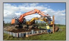
Plastic sheet piles are driven to define the perimeter of the bridge abutment. Log piles are driven to their full depth according to an engineered pattern using a side-grip vibro-hammer. The piles are capped with access mats, geotextile fabric and gravel to provide the bearing strength for the footing.
