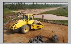
Plastic walls are anchored with tie-backs and reinforced with additional timber piles prior to compaction. The track dump, skid steer and compactors prepare the footing for the horizontally installed sheet pile bridge structure.
