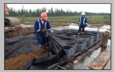
Access mats are used as a platform for the excavator to construct the first pier. The construction process is repeated using plastic sheet piling, wooden piles, fabric and compacted gravel. Steel ready rod is used in combination with steel channel to ensure the pier retains its shape.
