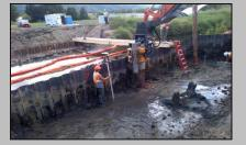
Silt curtains are installed to reduce sedmentation and a tarp installed under the old structure to catch debris during bridge removal. Steel sheet piles are driven to allow for footing excavation. The wooden work platform is supported by the sheet pile wall to provide workers access to both sides of the job site.
