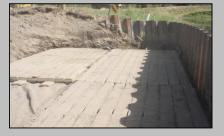
More than 100 fir-larch piles are driven to support the arch footing. Piles are cut even and a levelling course of sand is added. It is then capped with a 6" thick platform (access mat) and is covered with geotextile and gravel prior to footing placement.
