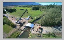
Concrete footings are placed on top of compacted fill. Cobble is positioned prior to the arch being installed. Successive crane lifts allow for the arch sections to be repositioned from the staging area and bolted to the footing plate as well as each other prior to torquing to design specifications.
