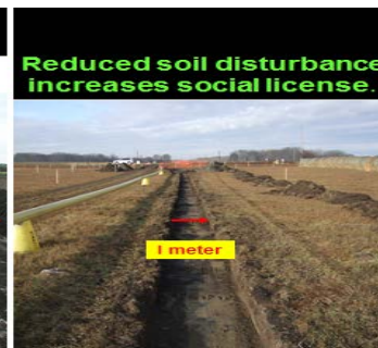
15 m soil salvage compared to 36" trench-line soil salvage
