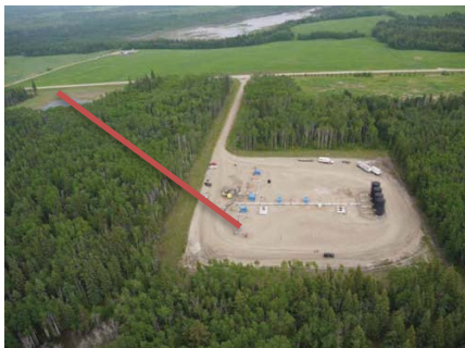
Pipeline installed – no disturbance!
