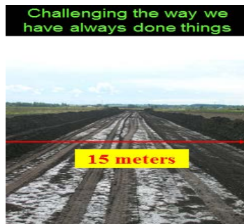
15 m soil salvage compared to 36" trench-line soil salvage
